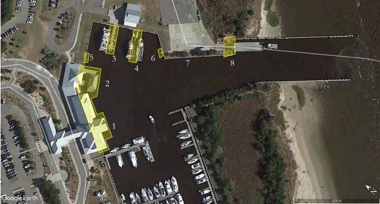
Facilities Inspected highlighted in yellow. Limits of Bulkhead Wall shown separately in
