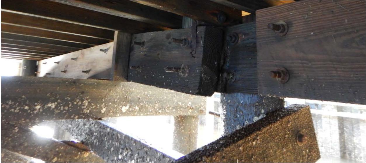
FIGURE 2-26: UNDERDECK VIEW OF TIMBER STRINGER
