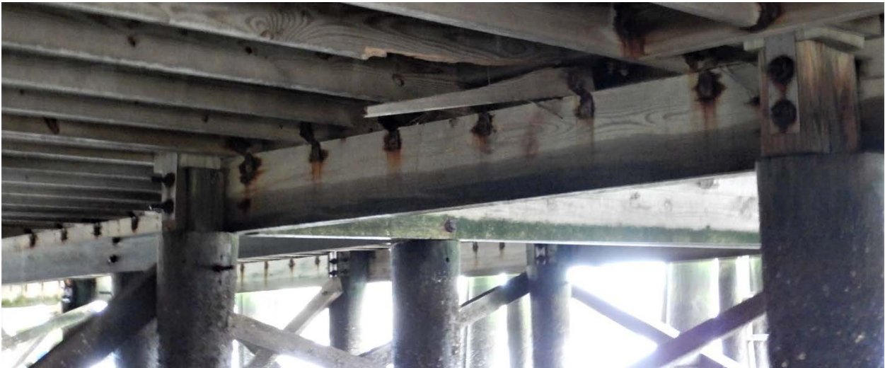
FIGURE 2-4: DPM B-GATE CONTRACTOR LANDING UNDER DECK FRAMING
