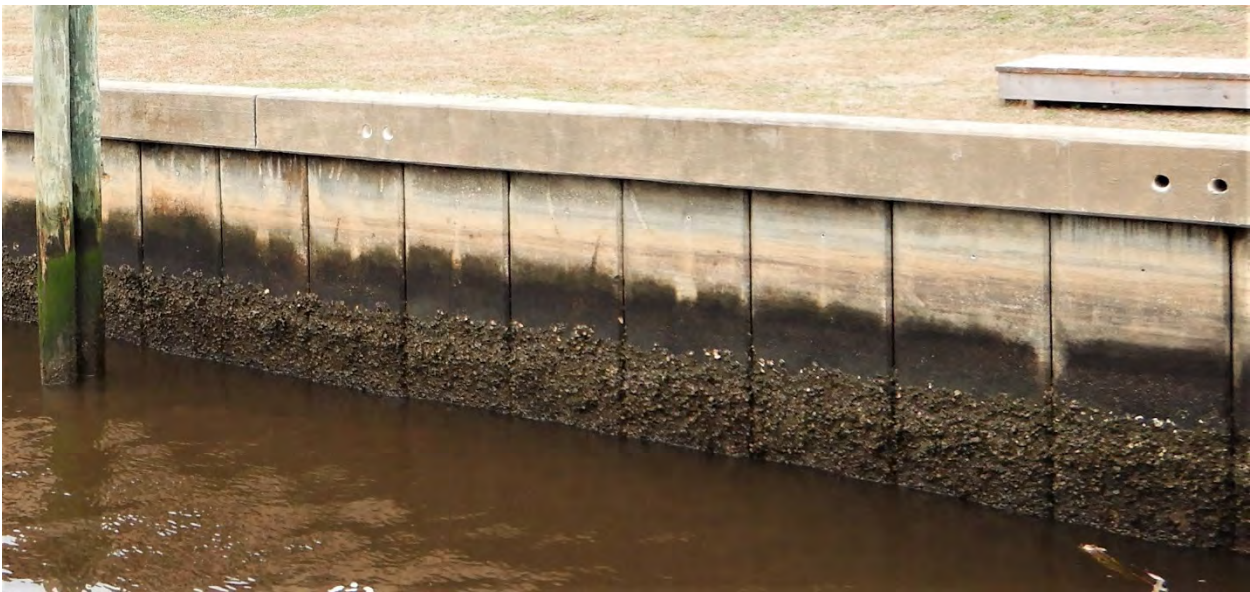
Location adjacent to "H" Berth and Maintenance Docks, looking West
