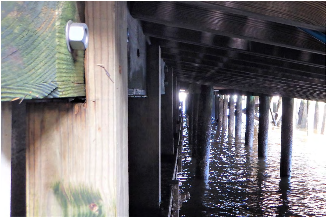
FIGURE 2-27: UNDERDECK VIEW OF CARGO RAMP
