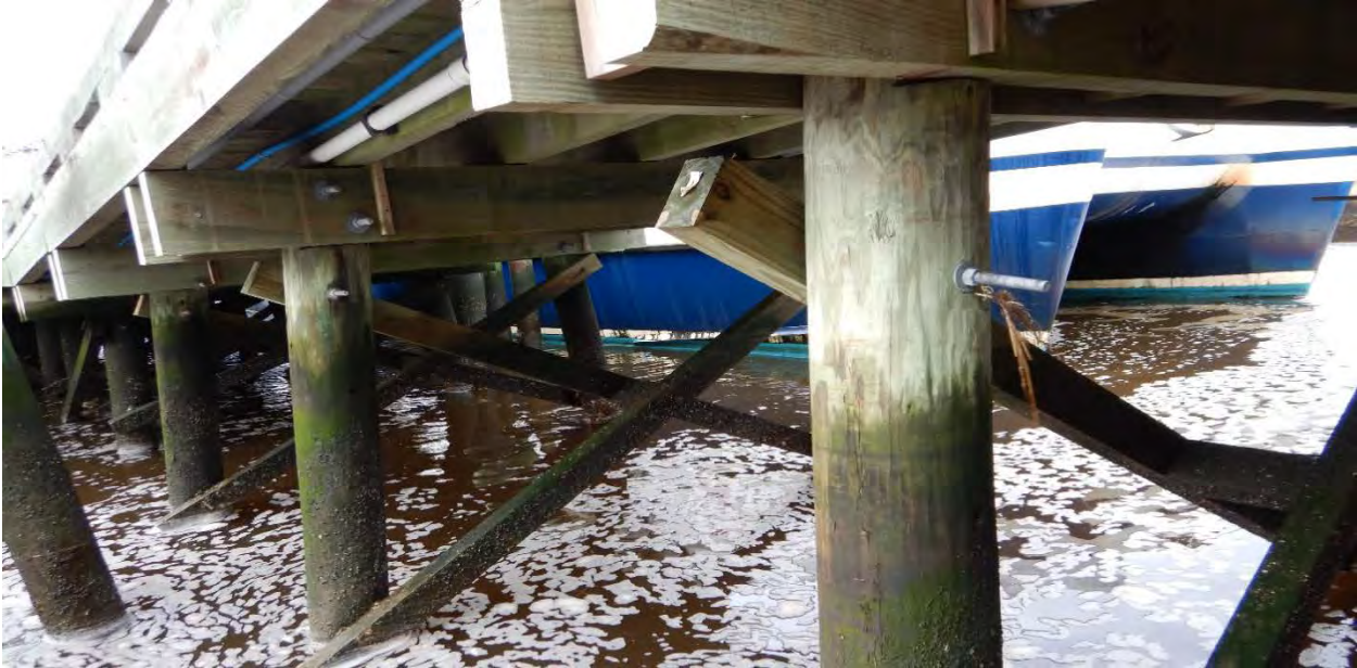
FIGURE 2-6: DPM MAINTENANCE FIXED PIER TIMBER PILE BENTS
