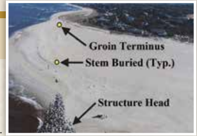
BHI's Terminal Groin — After successfully lobbying with other NC municipalities and coastal organizations for a state law to allow a limited number of terminal groins (now up to 6) in the state of North Carolina. BHI was the first to construct one in 2015/2016. (Photo from Olsen & Associates Monitoring Report No. 14).
